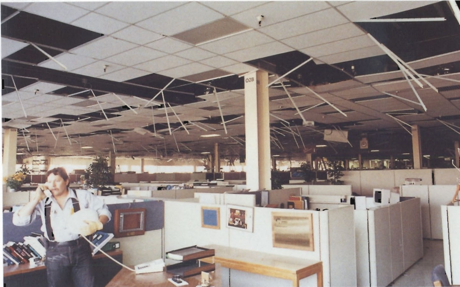
Ceiling tiles fell in many HP buildings during the quake. During cleanup at the Sunnyvale site, Jack Gephardt of facilities uses the phone of GM Bob Puette to make a report.
